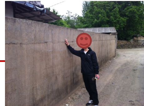
6. Too high wall
